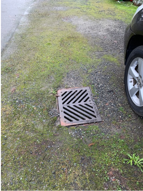
SE 27 th St. North Edge Catch Basin – Point E
