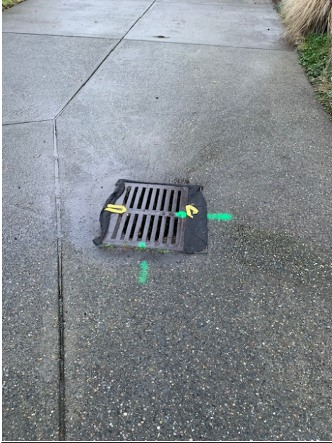
Catch Basin Point H driveway - West of 60 th Ave SE - Looking West
