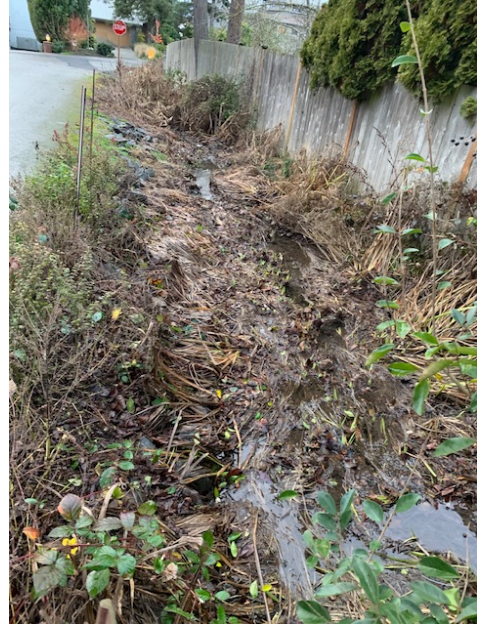
Open Channel Looking Downstream Point F
