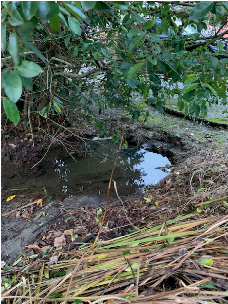
Culvert Discharge to open Ditch Point F
